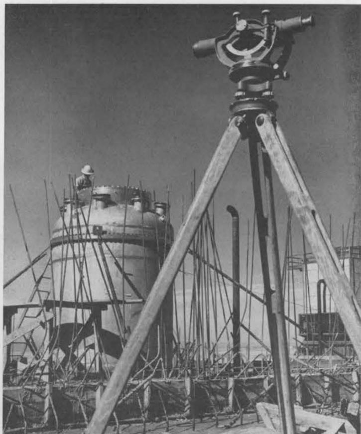
PRESSURE VESSEL of the Sandia Engineering Reactor Facility is shown in the maze of steel rods that will reinforce the concrete walls to be erected around it. The vessel will contain SERF's nuclear core. Access for the environmental materials testing programs to be conducted with the facility is provided by use of the underground chambers below the level shown by this photo.
